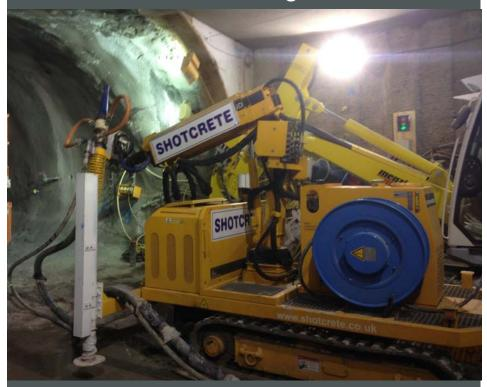
We were approached by the Main Contractor (BAM Nuttall and Taylor Woodrow) to assist them in overcoming the difficulties in constructing an SCL (Sprayed Concrete Lined) escalator tunnel.
